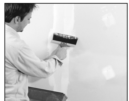
Figure 3.4: Tape and mud drywall
