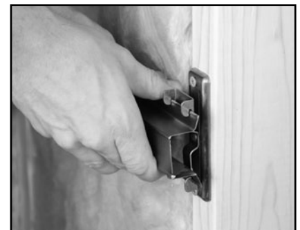
Figure 2.3: Snap QuietClip into hat channel
