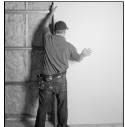
Figure 3.2: Install drywall vertically to hat channels
