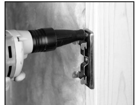
Figure 2.1: Screw QuietClips into stud wall
