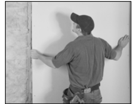
Figure 2.1: Install first layer of drywall
