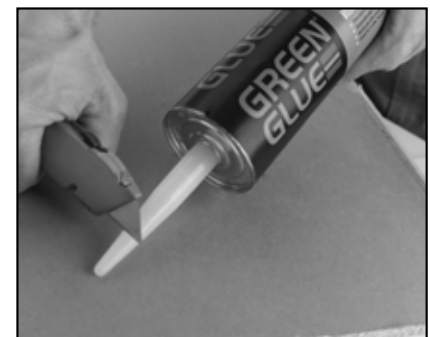
Figure 2.3: Cut a 3/8" opening in tube
