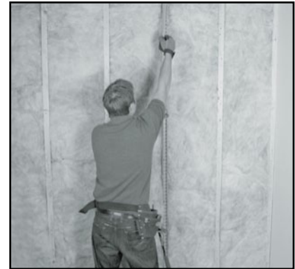
Measure the height of the wall
