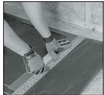
Cut Barrier to the appropriate length.
