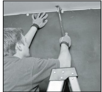
Fastener the barrier in 5 spot at top of roll.
